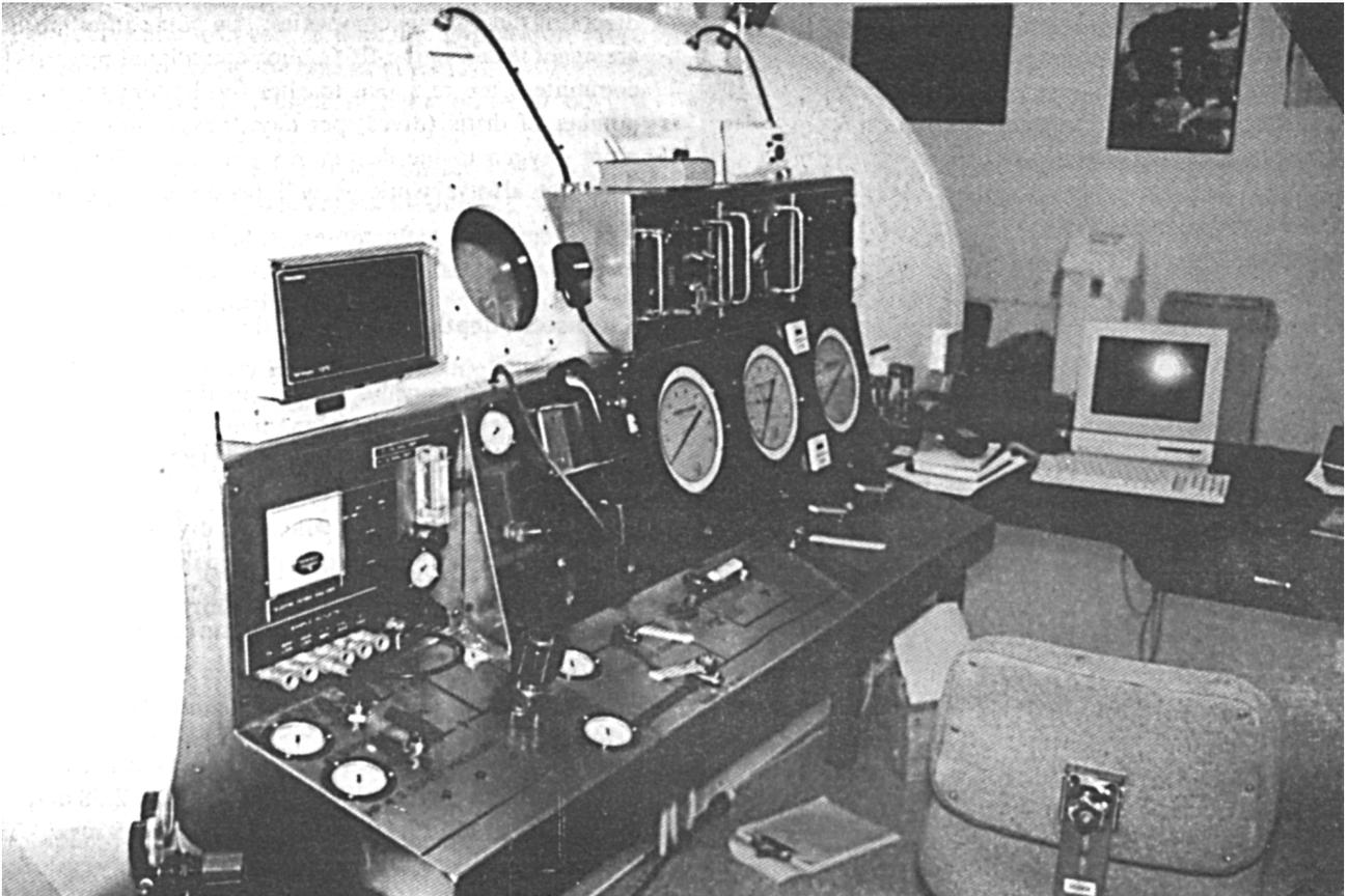
**Figure 1.** Side view of Broome recompression chamber
