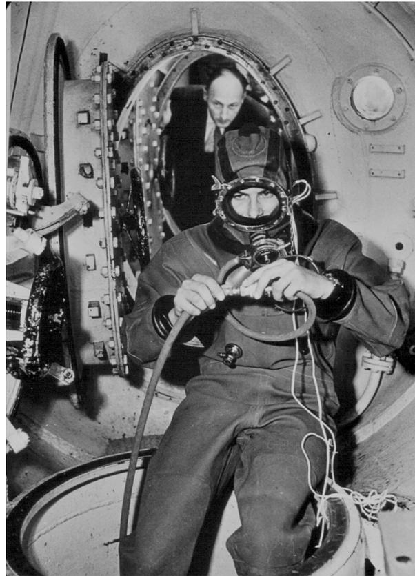
**Figure 2.** Hannes Keller (front) and Professor Bühlmann in the Toulon chamber before a 220 m chamber dive.
